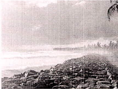
Figure 20:seawall made up of rocks in the Paravur in Kollam(kerala in India)
