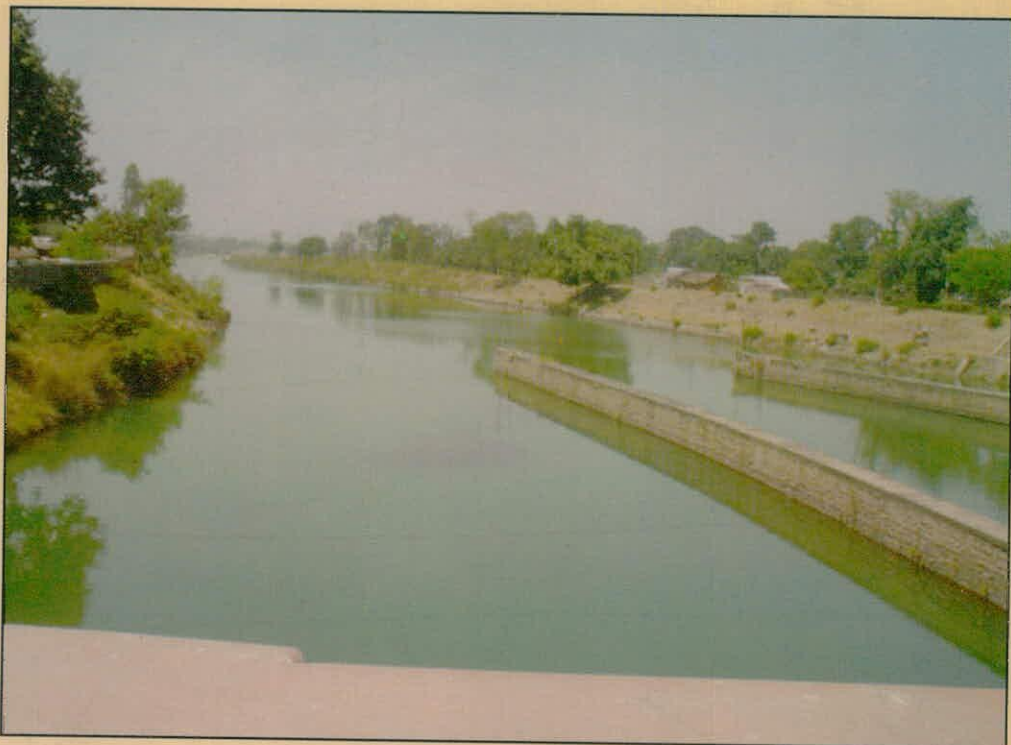
WYC near Hathni Kund Barrage
