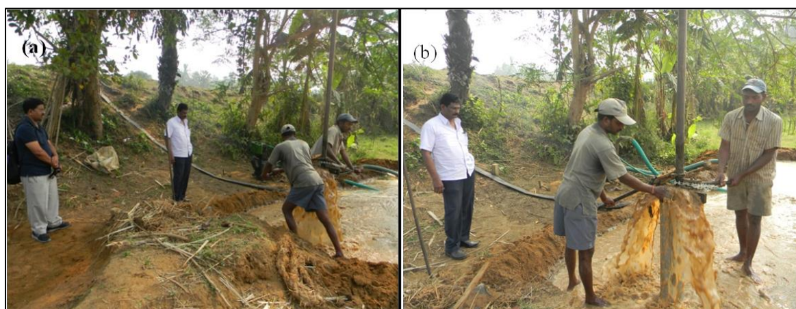
Photographs showing stages of drilling work in progress
