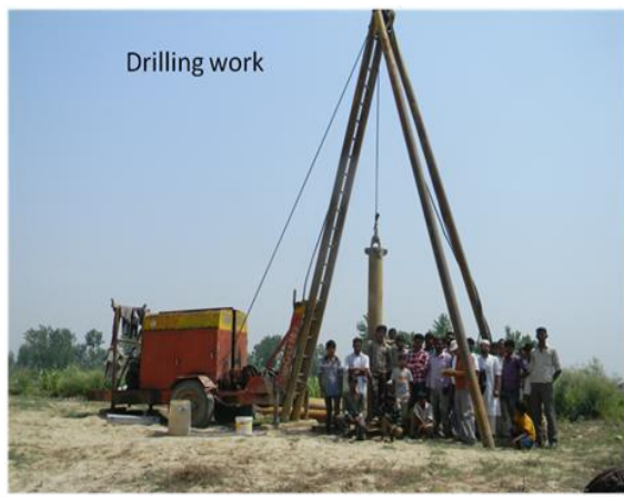
Photograph 1: Drilling work for RBF well RBF Development.
