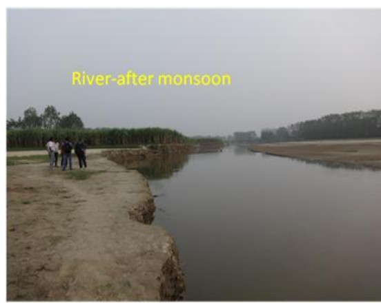
Photograph 2 : Dislocated riverbank of the site by erosion during 2016 flood.
