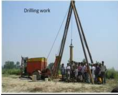
Photograph 1: Drilling work for RBF well Development.
