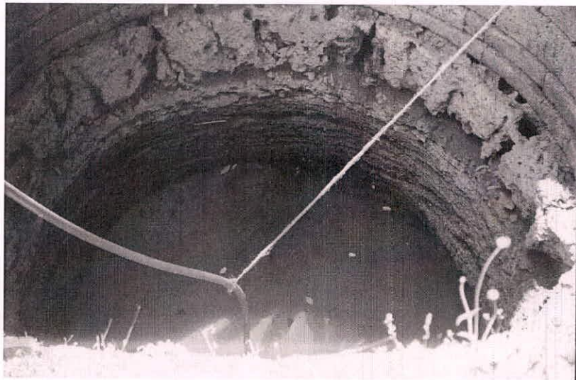
Fig. 5 Caverns in the upper portion of the calcareous sandstone horizon
