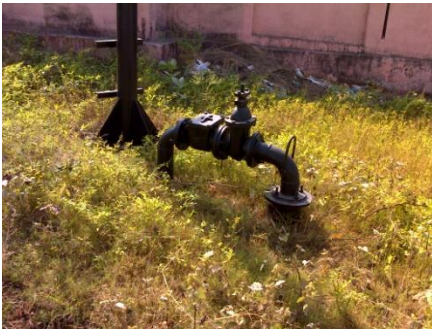
Infiltration well (TL 14) at Boria Colony
