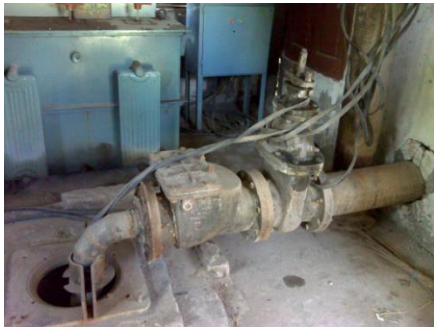
Infiltration well (TR 08) at M A Stadium
