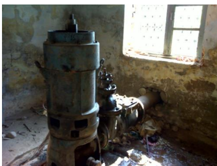
Infiltration well (TL 01) at Boria Colony
