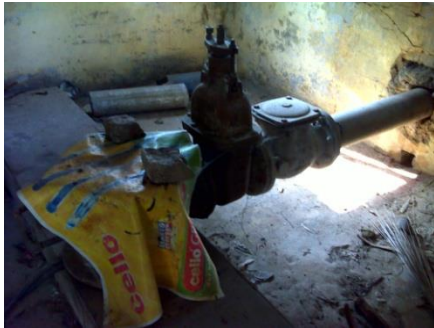
Infiltration well (TL 07) at Astro Turf Stadium, Jammu University
