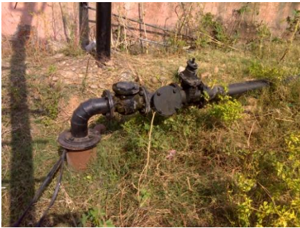
Infiltration well (TL 13) at Boria Colony
