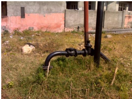
Infiltration well (TL 06) at Boria Colony
