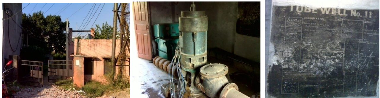
Infiltration well (TR 11) at Samadhia alongwith the Strata chart
