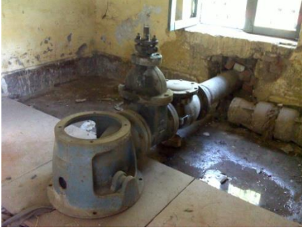
Infiltration well (TL 02) at Boria Colony
