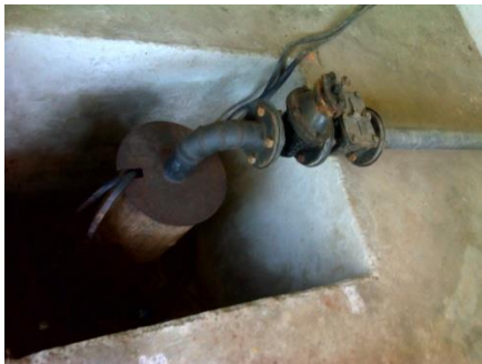
Infiltration well (TL 15) at Astro Turf Stadium, Jammu University
