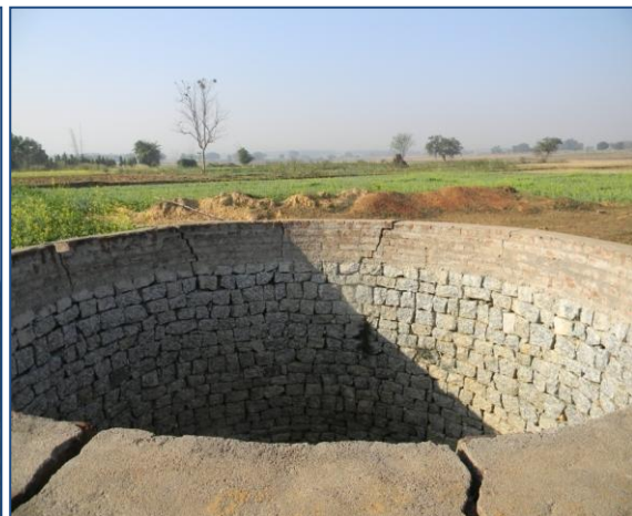
Figure 6: Dug well near the Kolsimri village being used for irrigation water supply.
