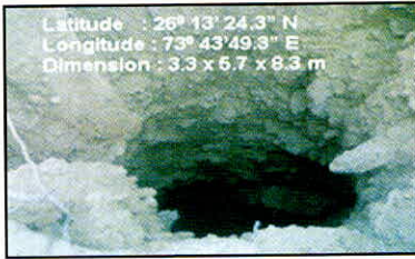
Sinkholes inside the reservoir
