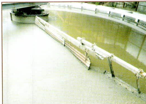
Malyana Sewerage Treatment Plant (STP)
