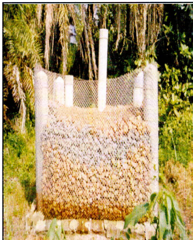
Figure - 2 Recharge well at Mopidevi
