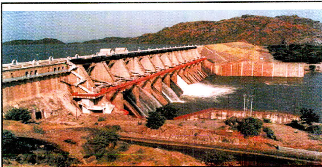
Figure - 1 A view of Dharoi dam in Sabarmati basin, Gujarat
