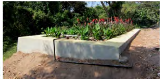
Fig 2: Photograph of HSSF-CW at IIT Bombay
