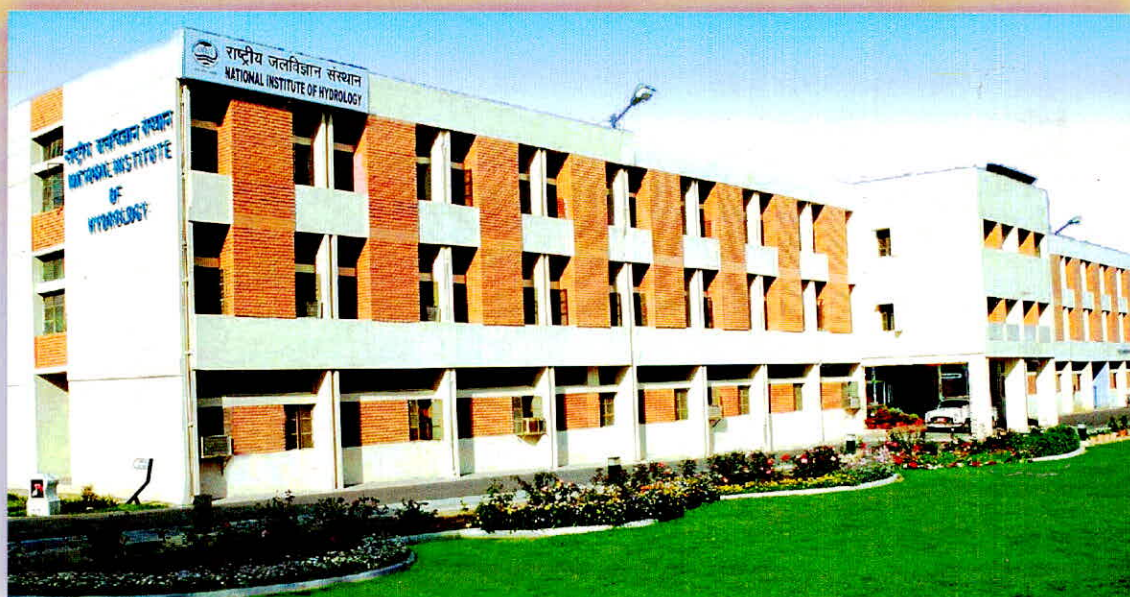
A view of NIH building at Roorkee
