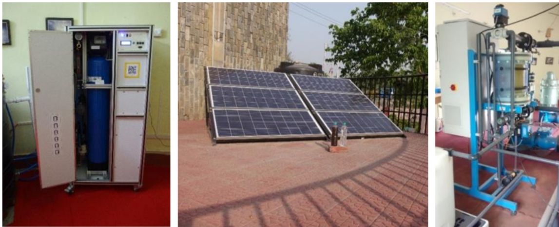
Fig. 4a–c Small- (left & center) and medium-scale (right) inline-electrolysis pilot plants at well 18 (Photos 4a & b: P. Otter, AUTARCON, 2016; 4c: Hydrosys / TZWD, 2016)
