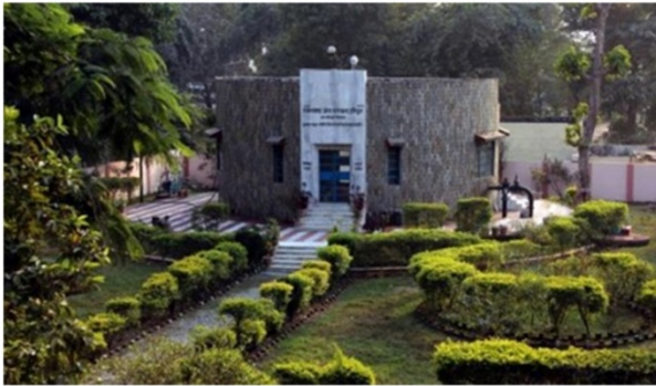
Fig. 3a RBF well 18 at demonstration site
