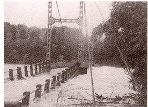
Fig. 3: Flow of river Sandai, Kagoshima, Japan during flood of 2006
