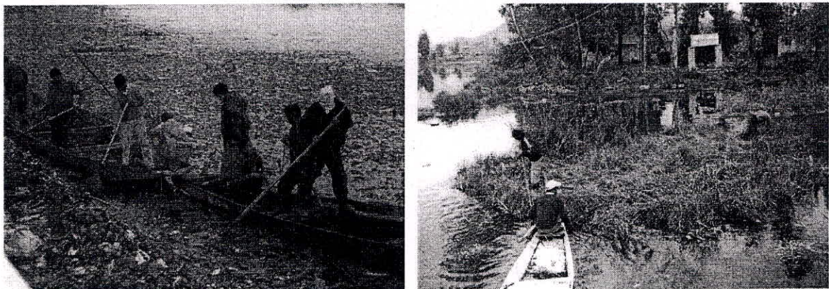
Fig. 15: Dredging/cleaning of Brari Numbal Lagoon
