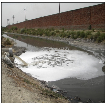
CETP Unnao Outlet into Loni Drain
