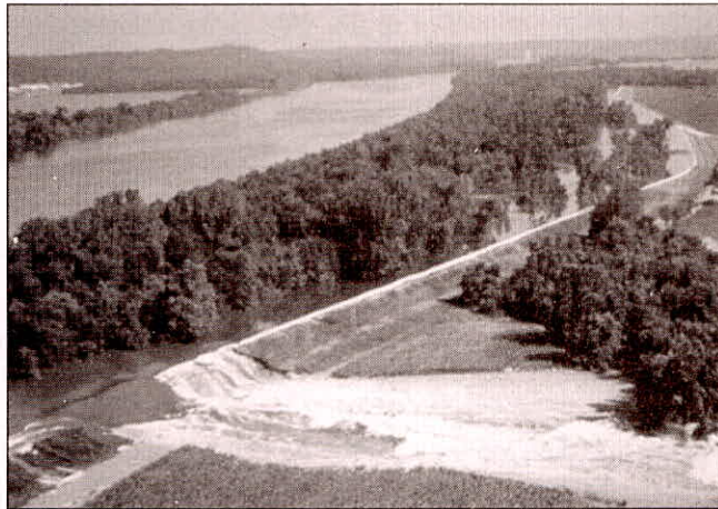
Fig. 3: A Levee Breach during the 1993 Flood, Photographs by the US Army Corps of Engineers
