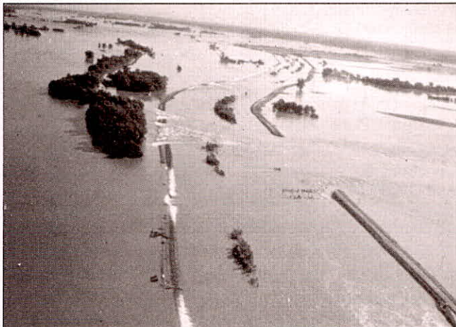
Fig. 4: Two Levee Breaches during the 1993 Flood on the Illinois River, photograph by M. Demissie of the Illinois State Water Survey
