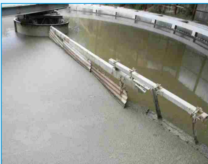
6 Malyana Sewerage Treatment Plant (STP)
