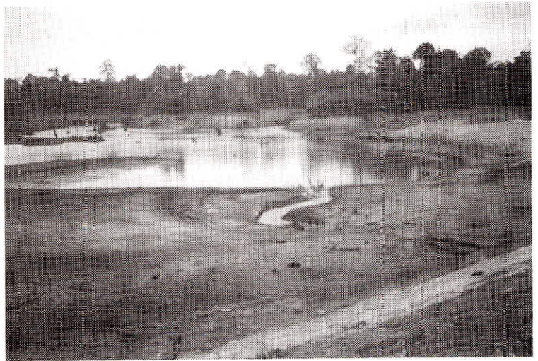
Fig. 24. State of R.K. Pur Dam, Little Andaman after 26.12.04 earth quake.
