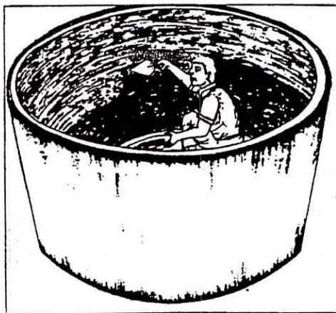
Figure 27 : Plastering inside tank wall
