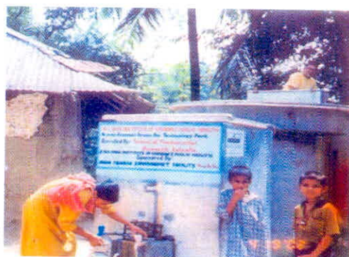
HANDPUMP ATTACHED ARSENIC REMOVAL PLANT-AIHH & PH
