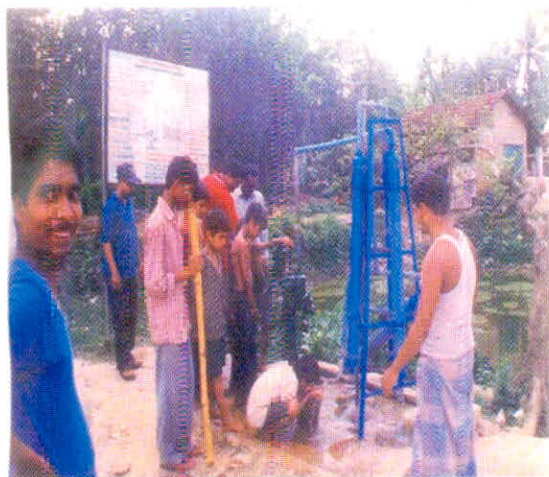
ARSENIC AND IRON REMOVAL SYSTEM-SFR MODEL
