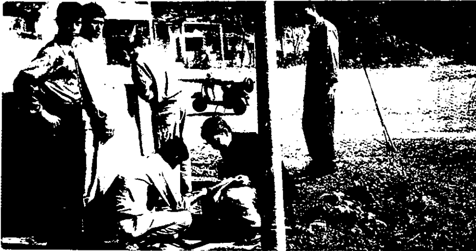
PLATE - II : SAMPLING & FIELD TESTING AT ZOO NARANGI SITE
