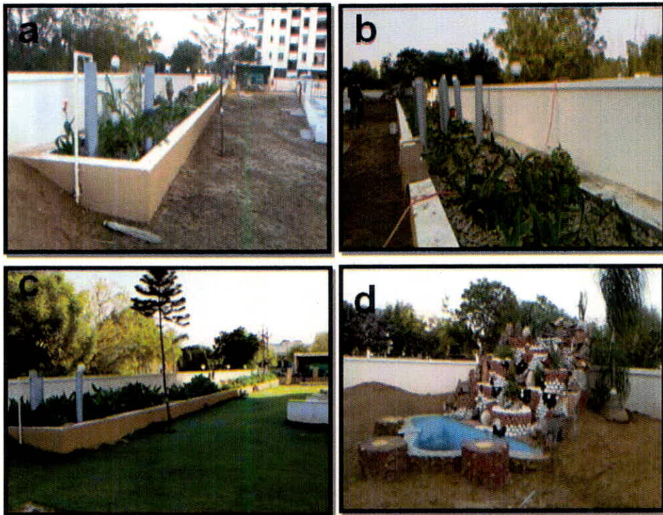
Figure 3.7: Pictures of Constructed Wetland, Jaipur, Rajasthan. (a) and (b) newly constructed wetlands, (c) working and maintained constructed wetland
