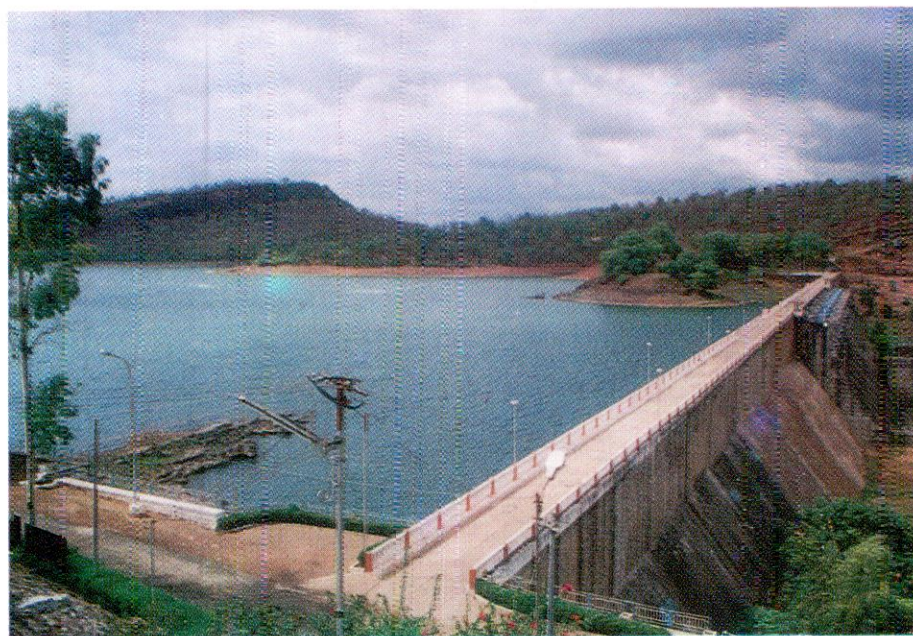
BARNA DAM (MAJOR PROJECT)
