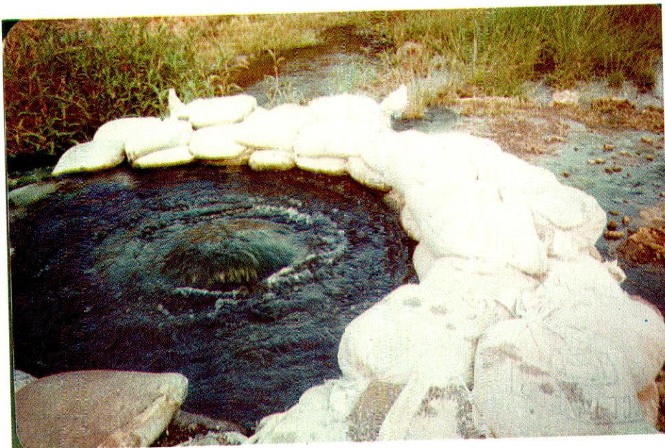
Isotope techniques can be used as a tool to study the nature of a boiling well due to leakage from a reservoir
