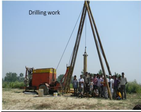
Photograph 1: Drilling work for RBF well Development.
