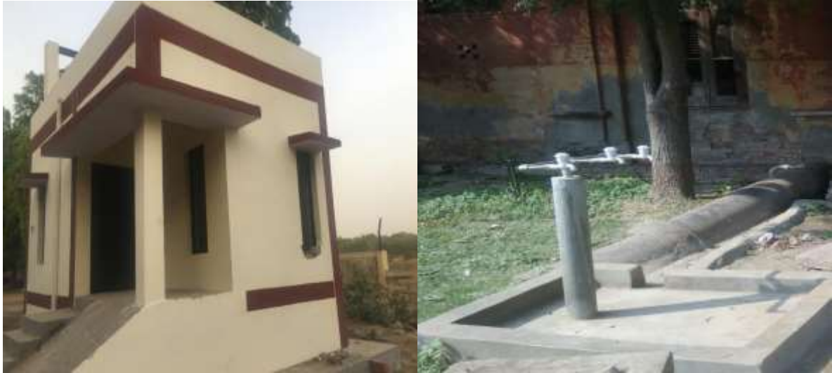
Developed pilot demonstration RBF scheme at Agra: (a) Pump House, and (b) Stand Post.
