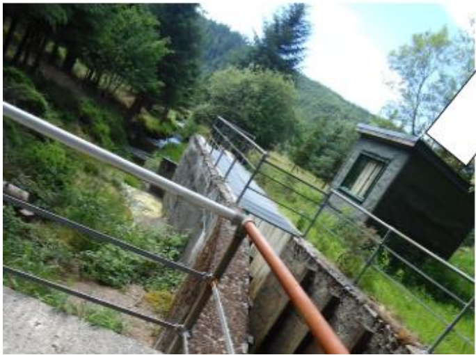
Gauging site 2 (Flume situated at large river bed slope)
