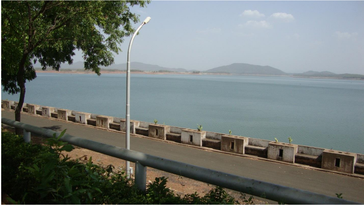
Tawa dam near Itarsi in Hoshangabad district, Madhya Pradesh.
