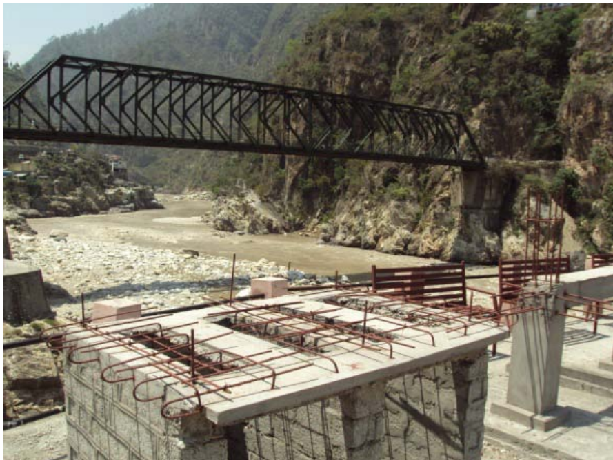
Fig. 13. Technology Park Under Construction
