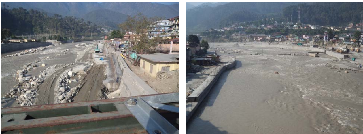
Fig. 3. River Protection Works of River Bhagirathi in Uttarkashi
