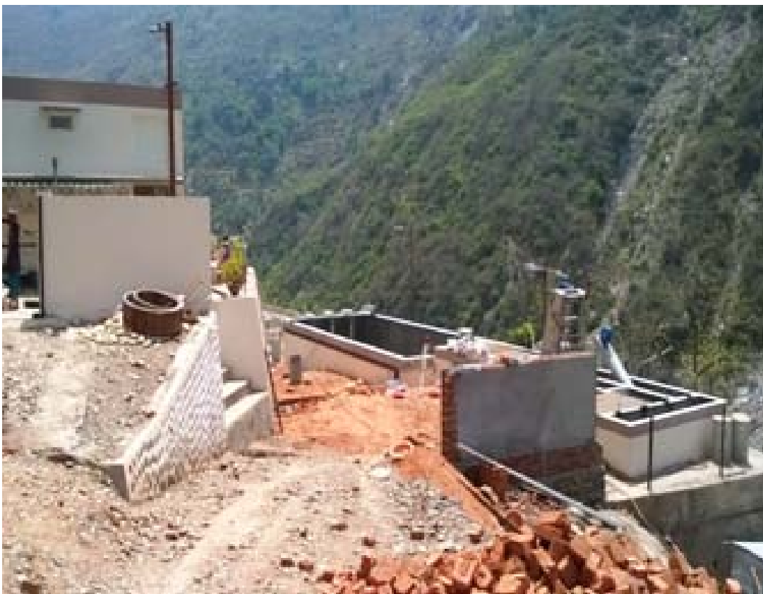
Fig. 6. Sewage Treatment Plant Under Construction at Devprayag
