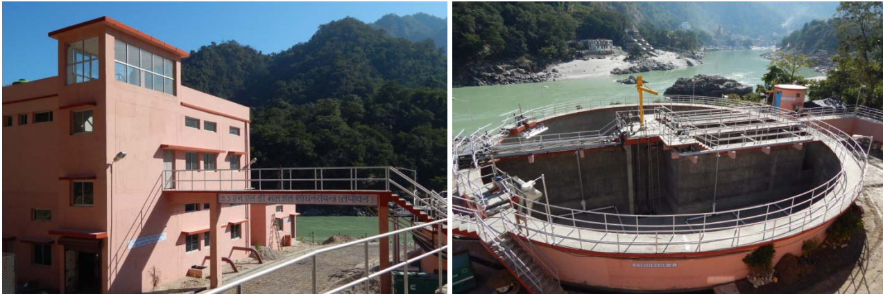
Fig. 2: Sewage Treatment Plant at Tapovan, Rishikesh
