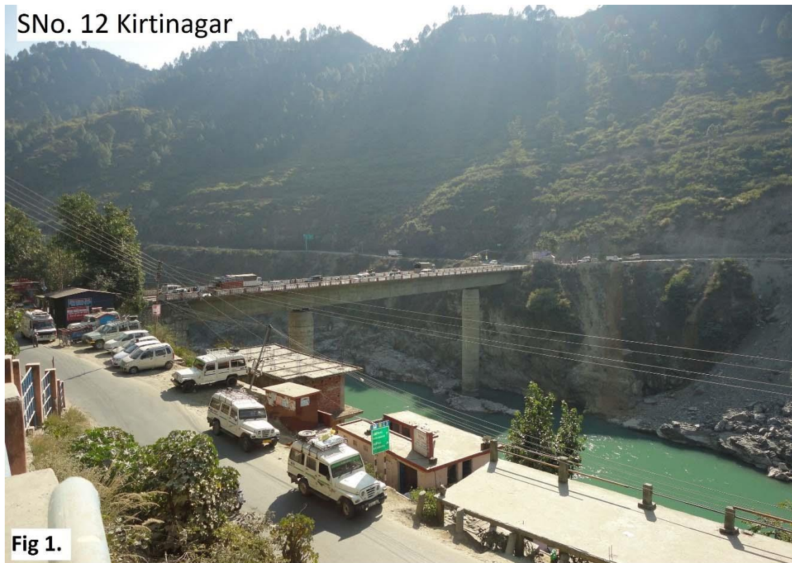
Location of New Bridge seen from Nagar Panchyat Kirtinagar
