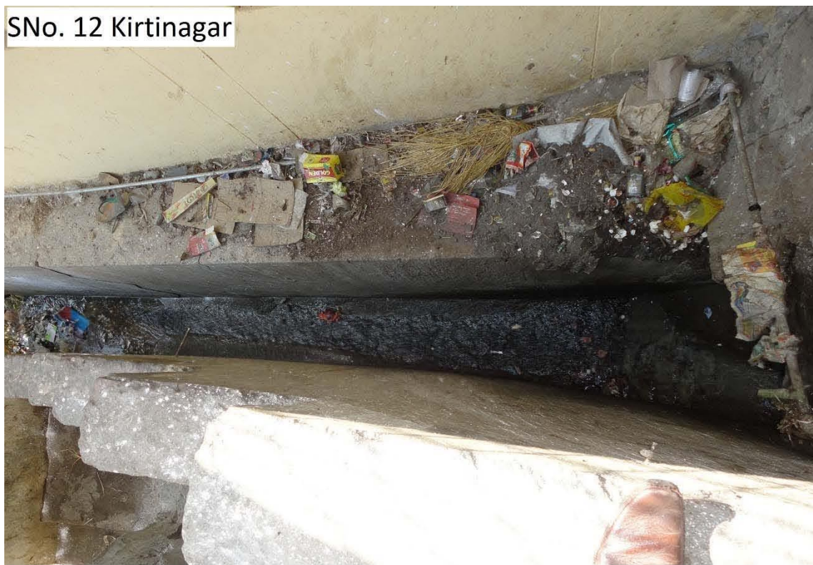
Fig 4. Open Drain 2 going into Alaknanda riverbed
