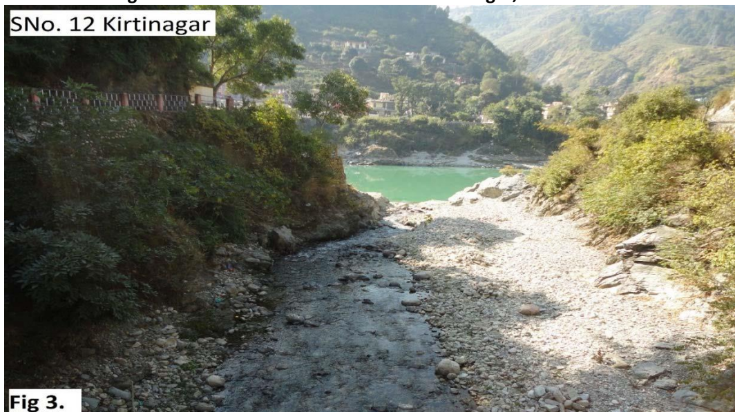
Dhundgad Stream Joining Alaknanda River d/s new bridge
