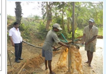
A photograph showing drilling of RBF well
