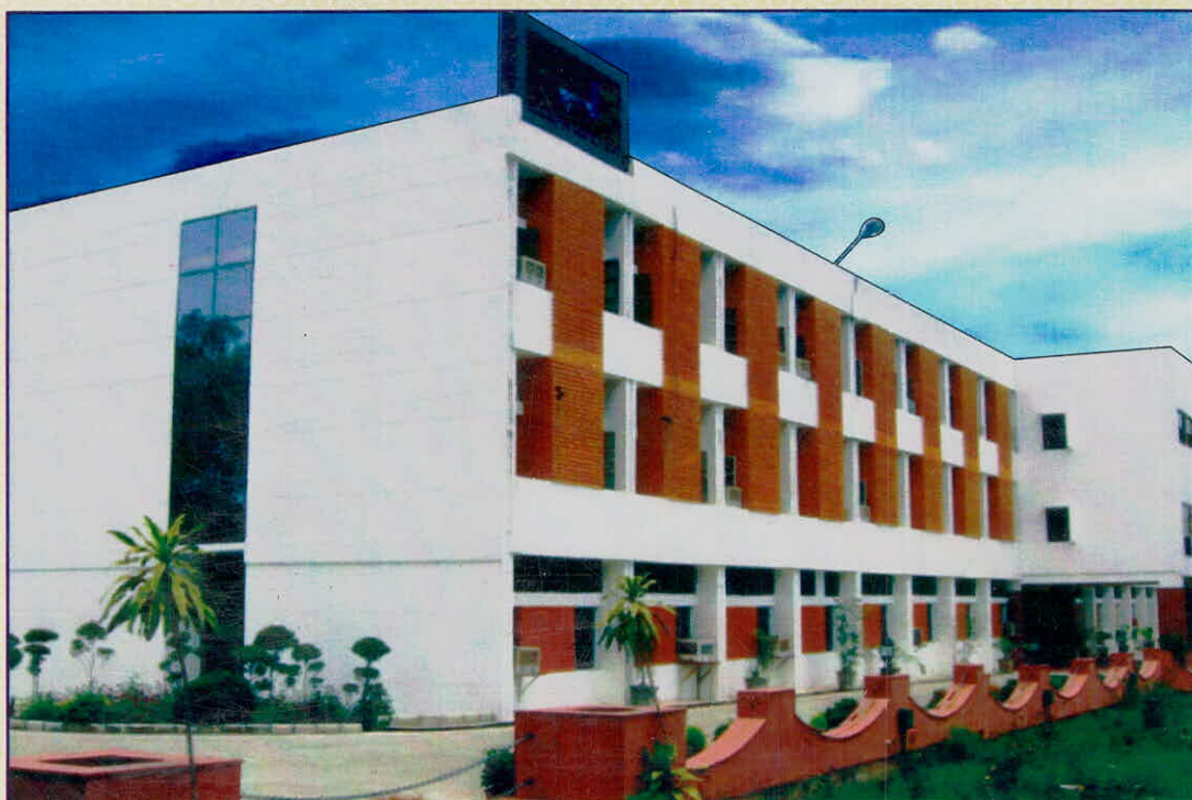
A view of NIH building at Roorkee
