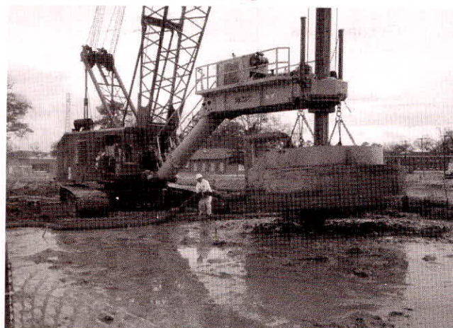
Fig. 4: ZVI-Clay Soil Mixing at the Site
