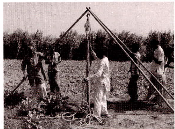
Fig. 3: Boring of piezometer
