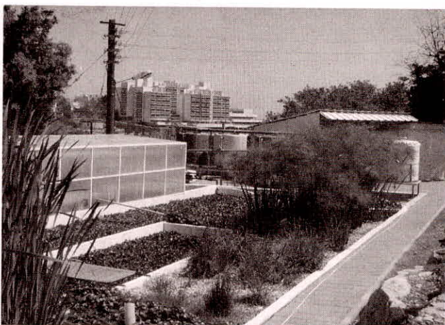
Fig. 9: Pilot for wastewater treatment by aquatic plants
