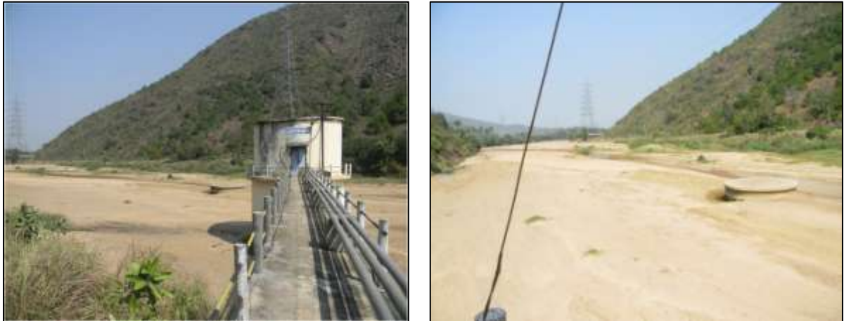
Figure 28: Intake Well constructed for water supply in the nearby villages at the upstream of the Varaha river and the dried up riverbed during lean period, which triggers a scarcity of drinking water supply during lean period (Feb.-May) in the villages. The upstream stretches of the river flows during monsoon period only.
