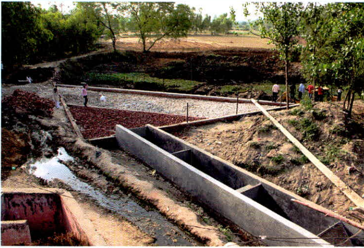
Fig. 1a: Constructed Wetland in village pond at Ibrahimpur Masahi
