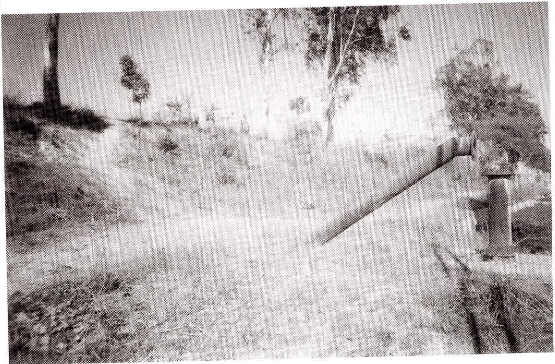
Fig. 3. Abandoned augmentation tubewell (by the side of augmentation canal) which was pumping water into the augmentation canal.
