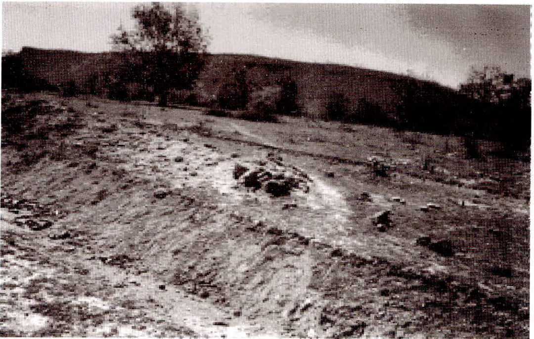
Fig. 4. Loose boulder check dam in Jharianala watershed, Tileijhar Village, Nawapada district.
