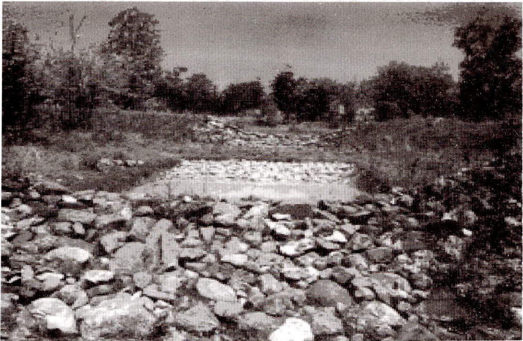
Fig. 3. Contour bunding in Jharianala watershed, Tilejhar Village, Nawapada District.
