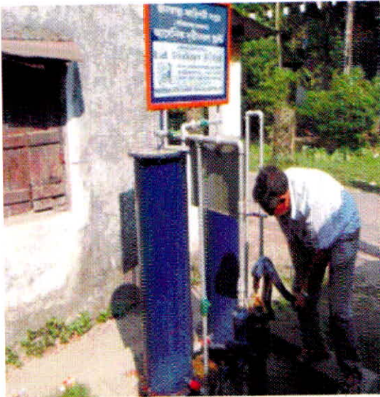
Figure 8.1 : Photograph showing a hand pump connected with Arsenic removal filter developed by M/s Pal Trockner Foundation Ltd, India, successfully operating under the community participation in O & M in Barasat, West Bengal.
