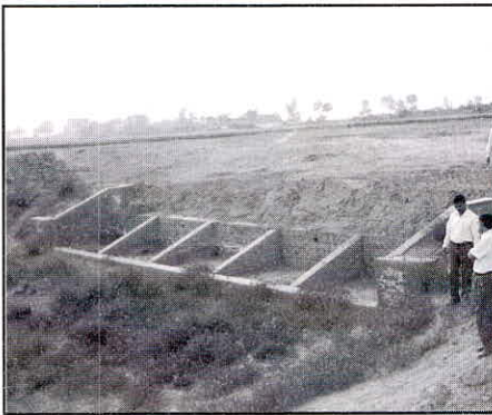
Fig. 2 : Masonary Drop Structure
