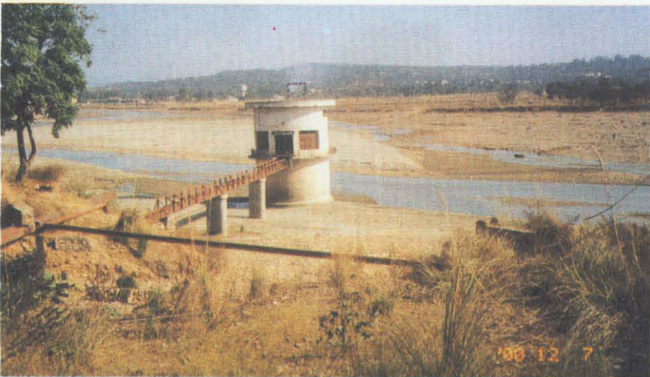
IIc Pumping station of the Basantar Lift Canal scheme, near Samba
