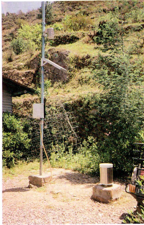
AUTOMATIC WEATHER STATION INSTALLED IN TEHRI WATERSHED, U.P.
