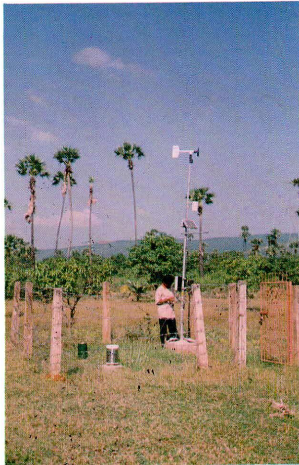
AUTOMATIC WEATHER STATION INSTALLED AT SANTI ASHRAMAM IN SUDDAGEDDA REPRESENTATIVE BASIN, ANDHRA PRADESH
