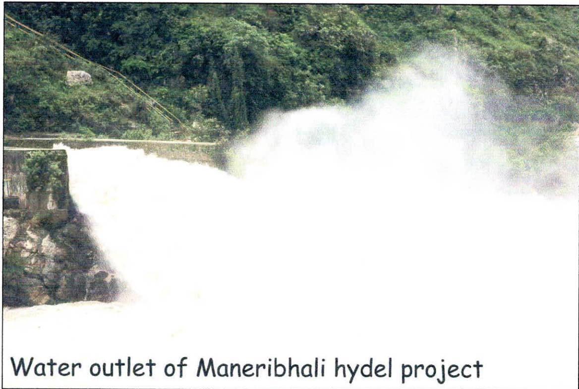
Plate 1.6 A view of Maneribhali Dam
