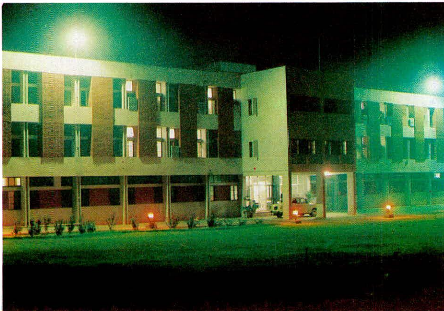
Front view of the Institute
