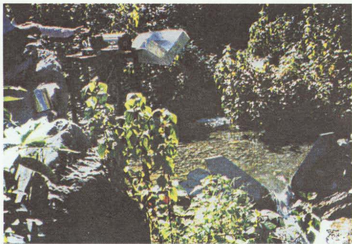
Plate II. Installation of water level (stage) recorder at Rumdhar
